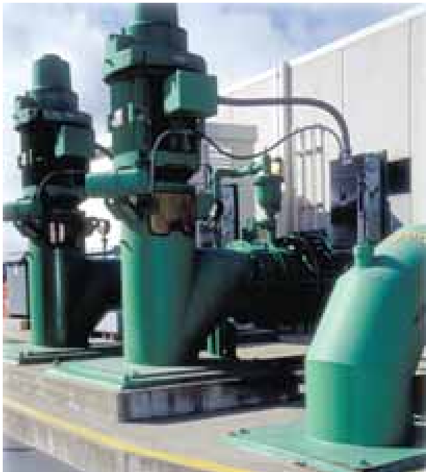
Typical vertical water pumps
